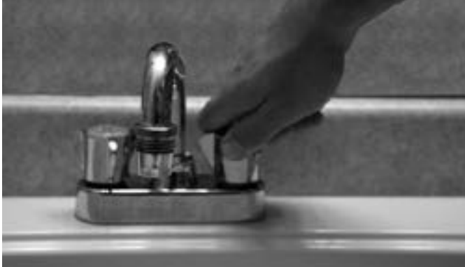
8. Open nearest faucet to relieve pressure and drain plumbing lines.
