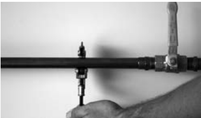
9. On a new installation not already plumbed for a water softener, cut out section of main water supply line downstream from the supply shut off, at position softener is to be installed.
